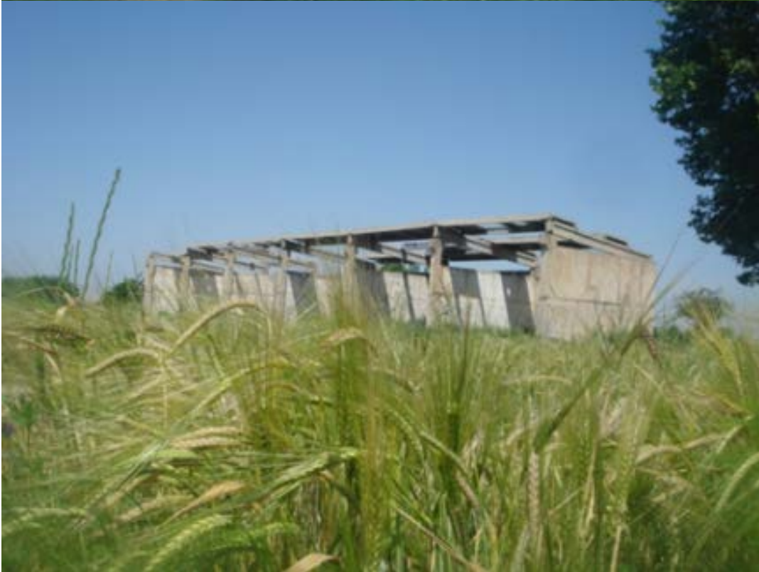
Figure 5. Typical former warehouses for storing pesticides
